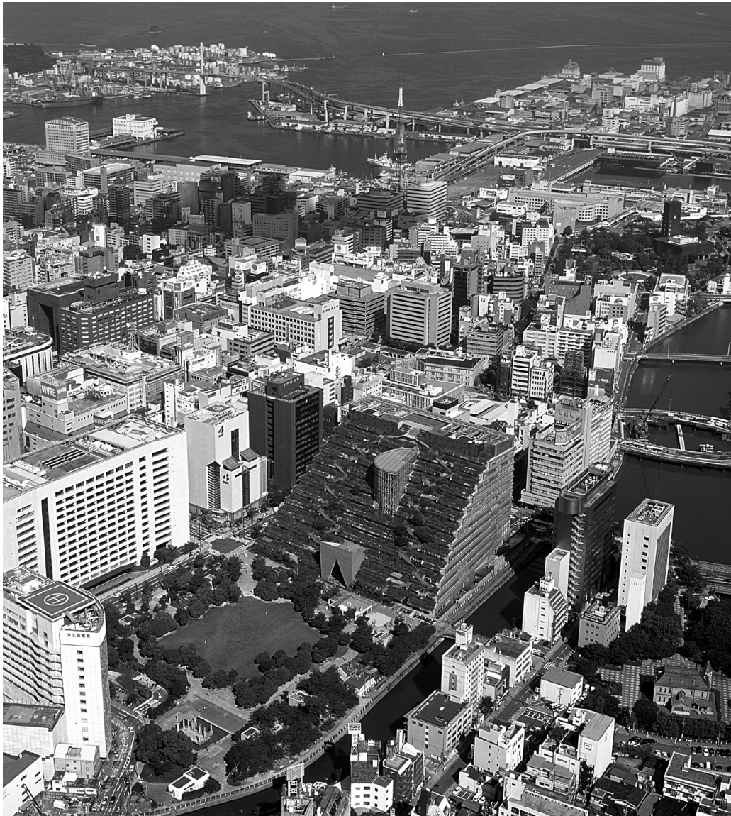
Emilio Ambasz & Associates, Fukuoka Prefectural International Hall, 1995. Photo: Hiromi Watanabe – Watanabe Studios.
