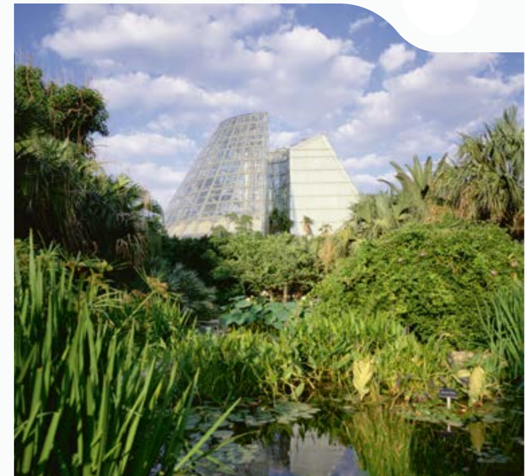
In the hot, arid climate of southern Texas, greenhouses need to keep out the sun as much as let it in. For Emilio Ambasz & Associates's award-winning 1982 Lucile Halsell Conservatory in San Antonio, Ambasz "used the earth as a container" to control light and heat while minimizing the need for mechanical systems, reducing building costs by 20 percent.
